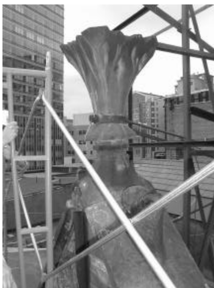
Detail of the significantly-deteriorated top of the pedimented gable, in the midst of its removal
