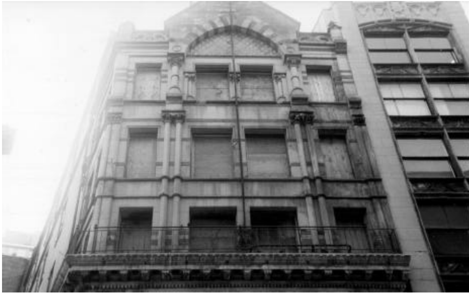
Detail of the front façade, including the arched top of the pediment that was removed
