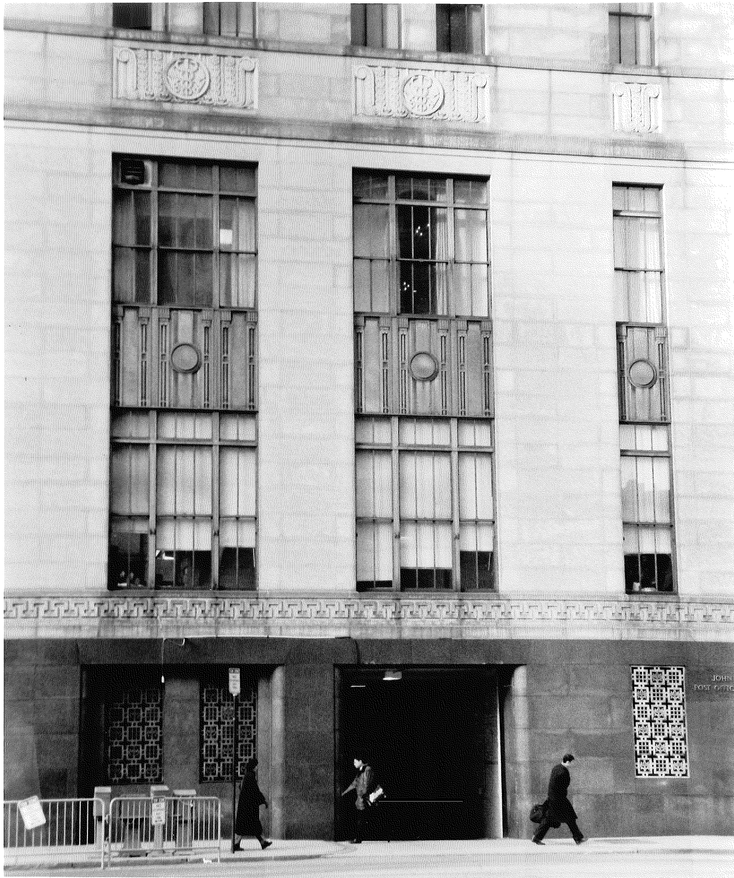
John W. McCormack Post Office and Court House Post Office Square Elevation (detail: water table, aluminum spandrels, grills, and sash) Photo Credit: Boston Landmarks Commission, 1997
