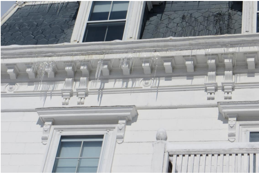
Detail of façade cornice with brackets and molding
