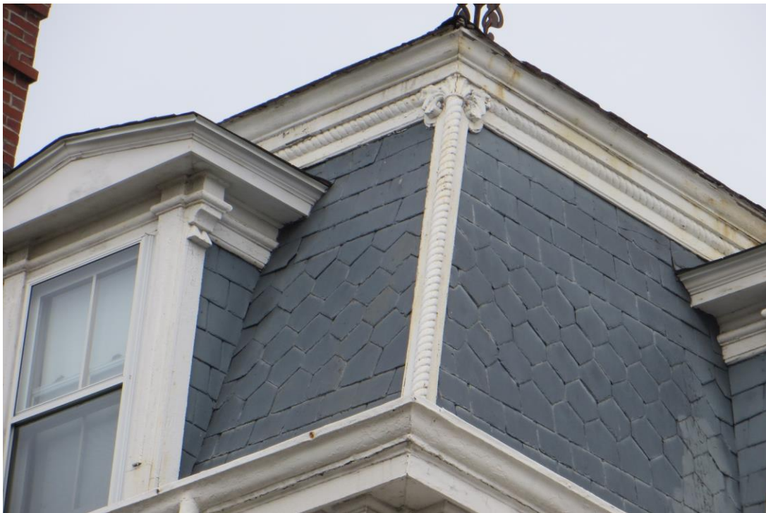
Rope molding and patterned slate on mansard roof - southwest corner
