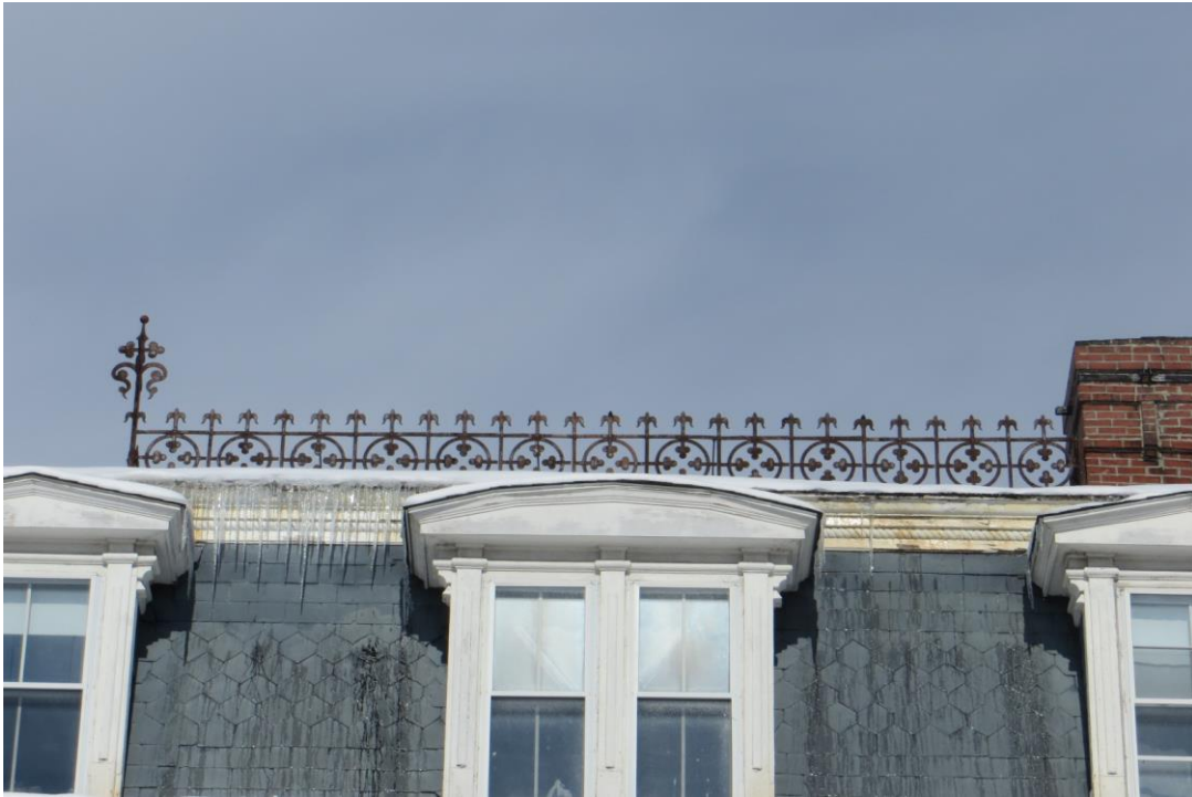
Cast iron cresting on roof
