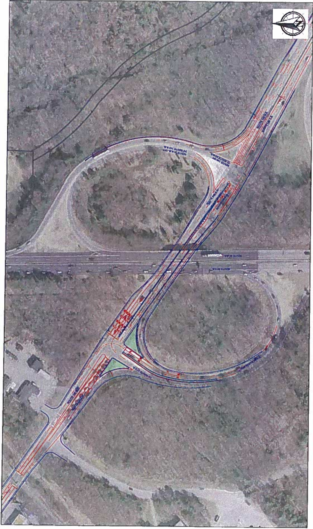
Figure C-1. Route 24 NB and SB Ramp (Exits 12A and 12B)/County Street (Route 140) Interchange
