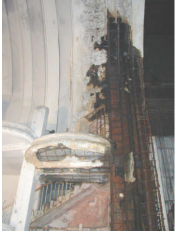
Detail of the proscenium arch showing the deterioration of the plaster (right)
