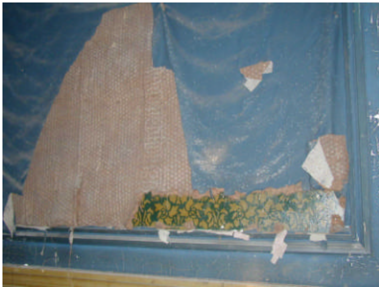
Detail of the matting added (left) to improve acoustics, probably 1930s or 1940s
