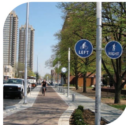
Special paving separates the at-grade bike path from the sidewalk, improving safety for walkers and bikers.
