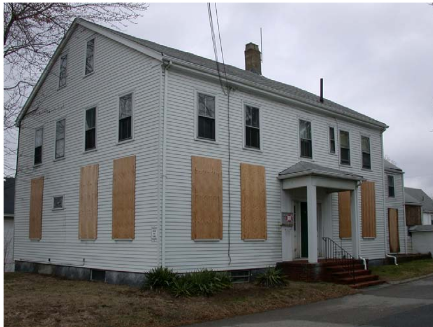
View from southwest.
