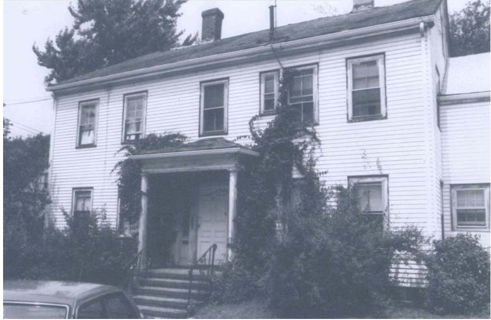
Sparhawk House at 45 Murdock Street, taken about 1979 with porch and entrance intact.
