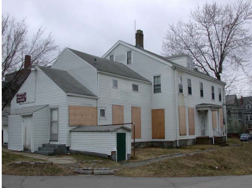
View of house from northeast.
