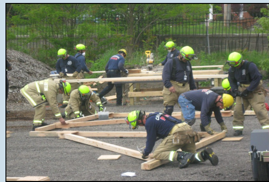
Members of regional fire departments work to secure exterior shoring during Urban Shield.
