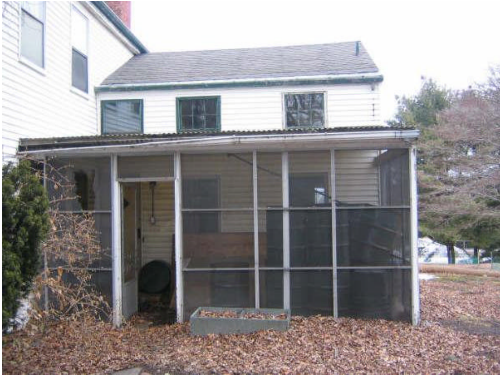
Screen porch addition to the ell. (BLC staff photo March 2007).
