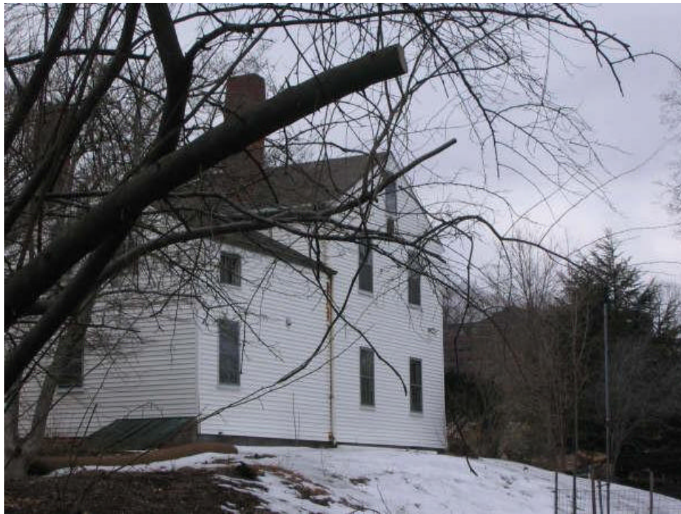
Northern elevation of the Lewis-Dawson Farmhouse. (BLC staff photo March 2007).
