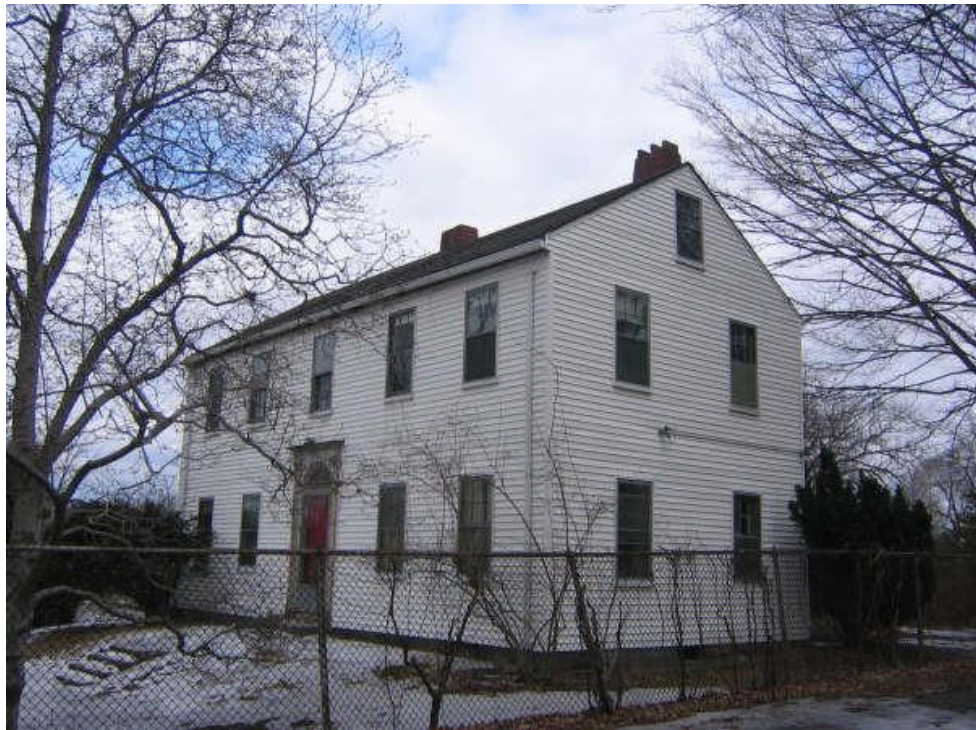
Western and southern elevations of the Lewis-Dawson Farmhouse. (BLC staff photo March 2007).
