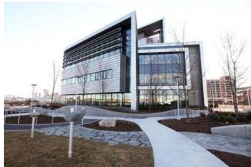
The Spaulding Rehab Hospital was built high above the floodplain with the mechanical suite on the roof. This reduces pollution and contamination caused by storm surges.
