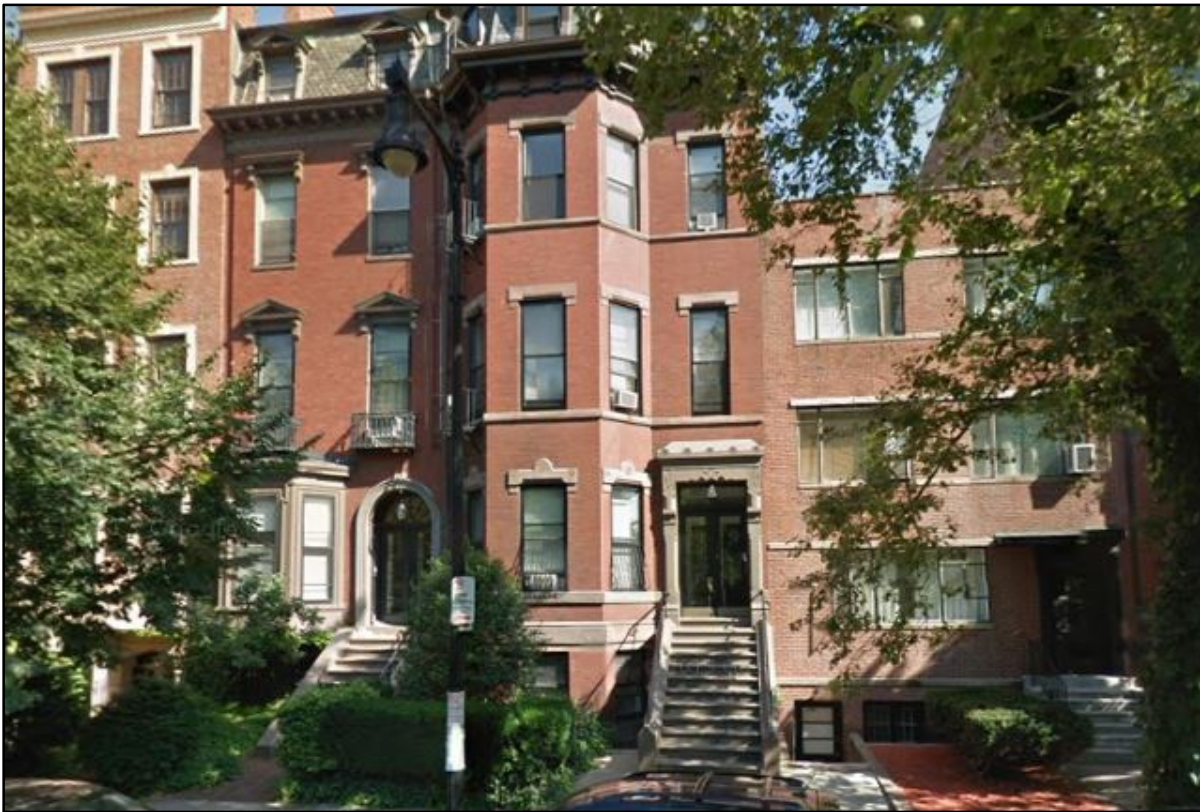
Photo 1. The fire building is the one with the bay windows from the basement to the fourth floor. The entrance to the basement apartment is under the steps.
