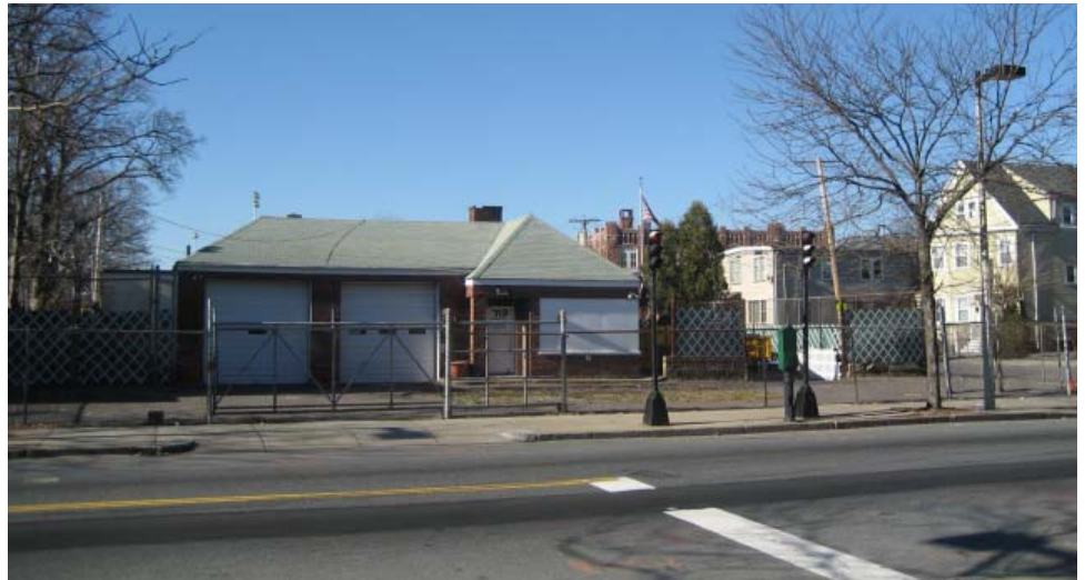
Existing structure at 719 Washington Street
