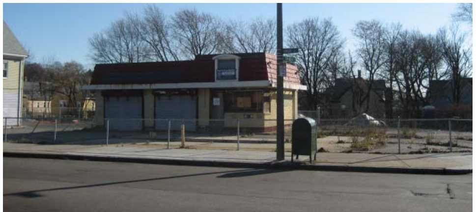
Existing structure at 191 Bowdoin Street
