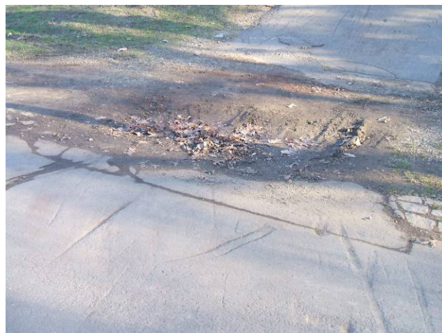
Figure 15. Along Tremont Street
