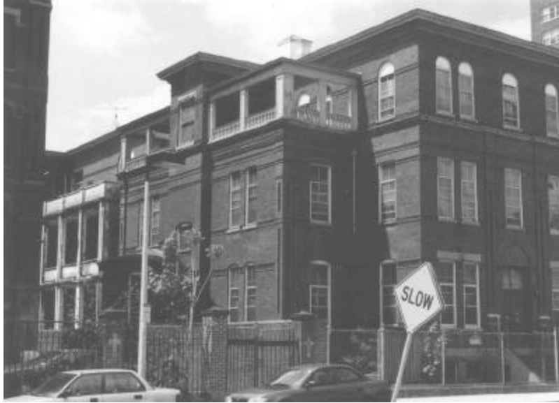
¾ view of the convent building from Smith Street
