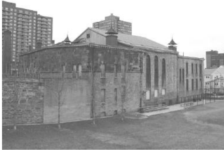
East façade and rear of St. Alphonsus Hall from the adjacent baseball field
