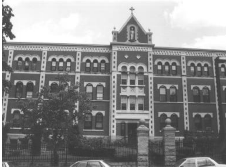
Front façade of the rectory (Tremont Street)
