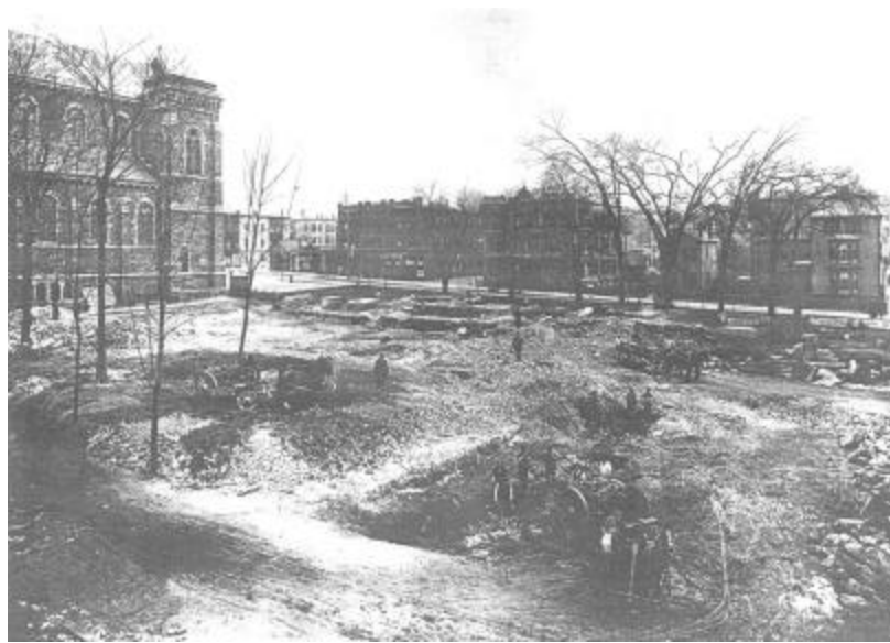
Construction of the rectory building
