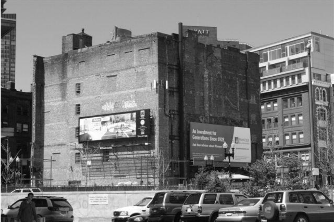
South and east elevations of the building. (Photo: Wendy Frontiero, May 2007).
