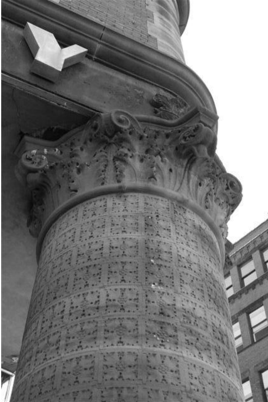
Column detail, corner of Kingston and Essex streets. (Photo: Wendy Frontiero, May 2007).
